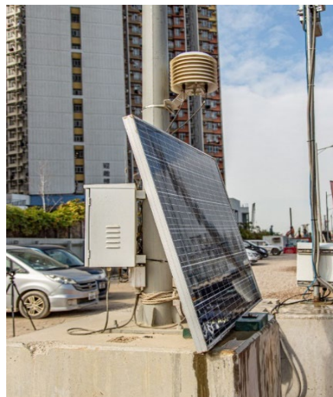
於主地盤通道應用太陽能板作照明 Installation of solar panels for energy supply to lightings along the main site access
