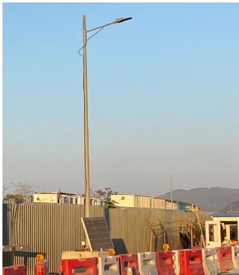
於主地盤通道應用太陽能板作照明 Installation of solar panels for energy supply to lightings along the main site access
