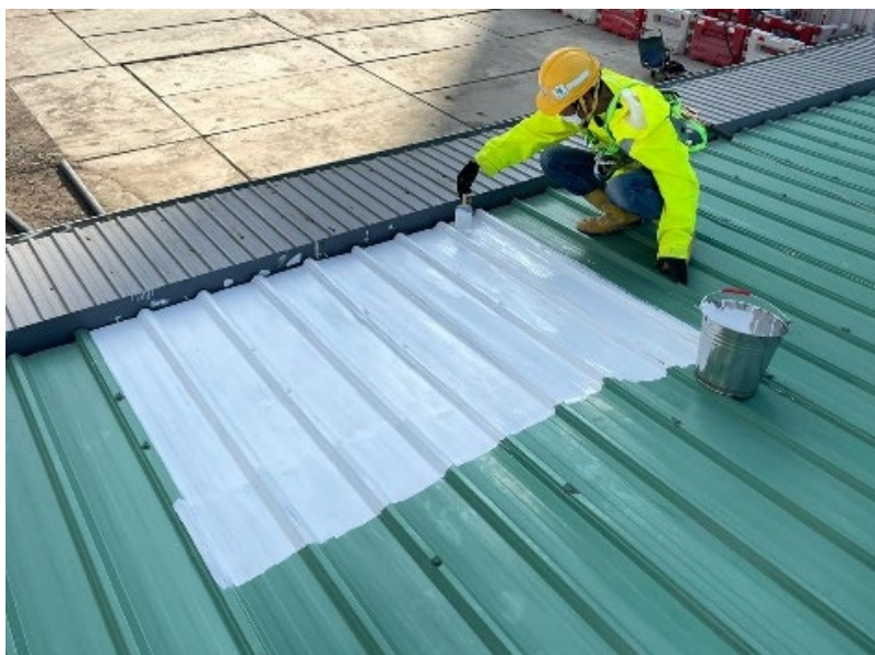
於地盤辦公室應用被動式輻射製冷塗層 Adoption of passive radiative cooling paint at the roof of site office
