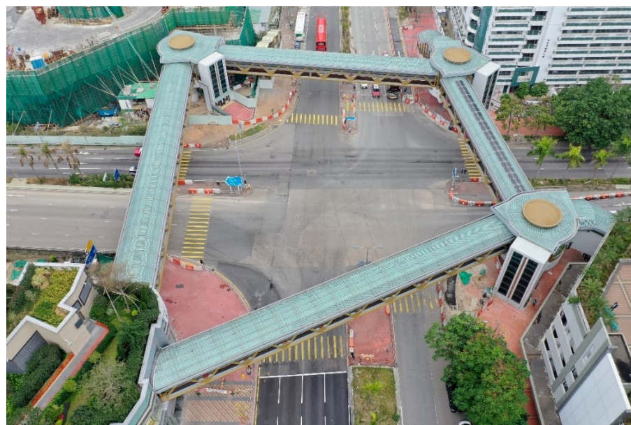
地盤和行人天橋裝設太陽能燈作夜間照明 Solar lights at works area and footbridge
