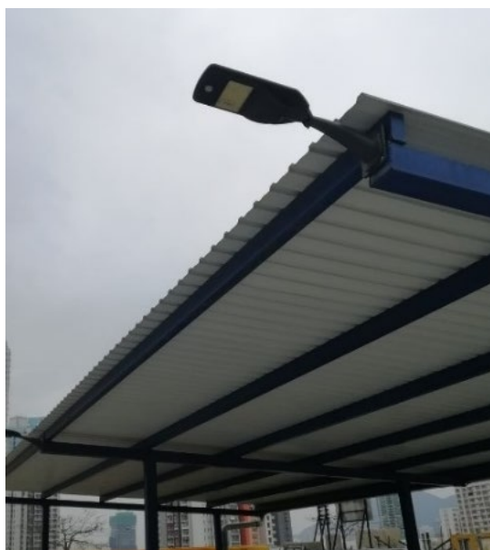
於主地盤通道應用太陽能板作照明 Installation of solar panels for energy supply to lightings along the main site access
