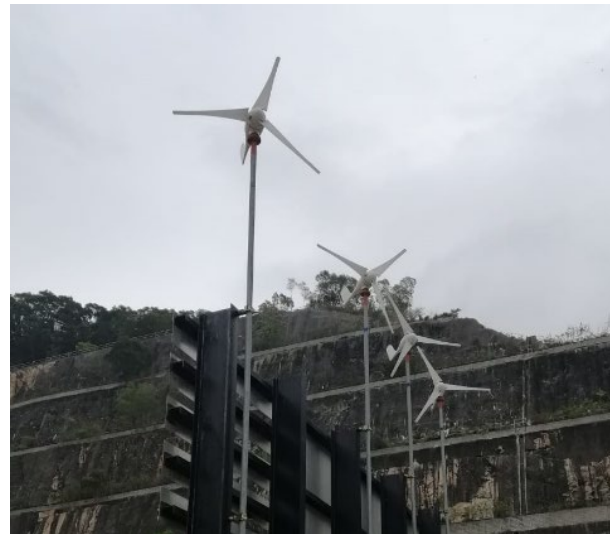
於地盤採用風力發電機 Installation of wind turbine at works area
